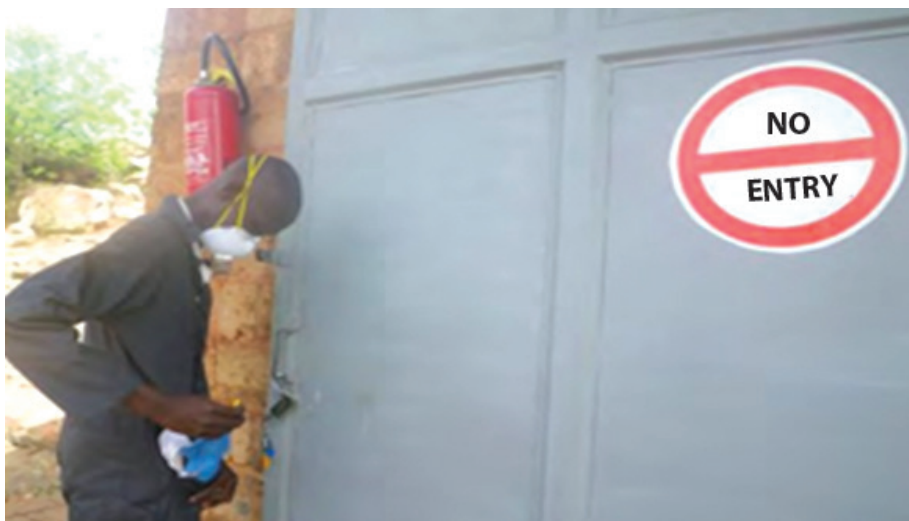
Fig 10.5: Storage facility with lock, fire extinguisher and warning sign
